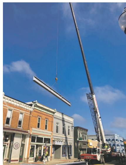
Steel columns supporting the Williamston Theatre's new, pole-free superstructure were swung into place in August of this year.
